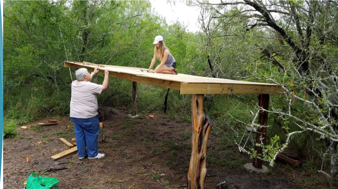
Photo blind building in progress. © Brian Loflin
